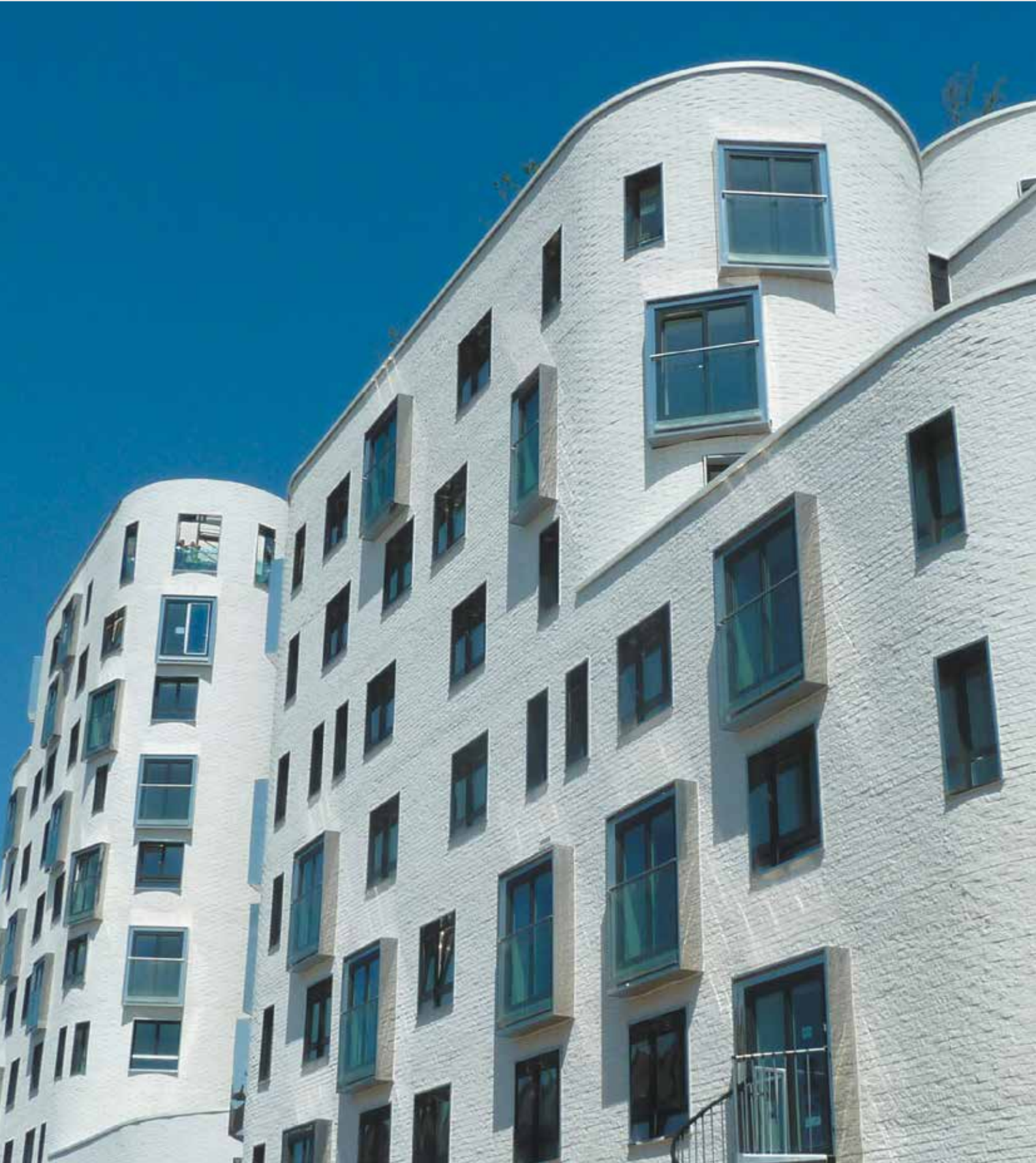
Woningen Clapham One PPP, Londen (UK) ▼
